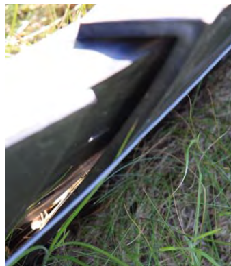
Fig. 34: Defective amphibian fences
