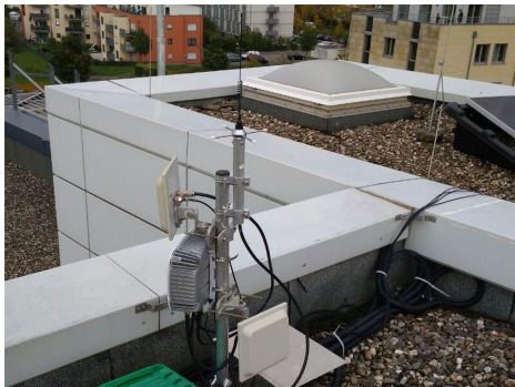
Fixed LoRa transceiver.
