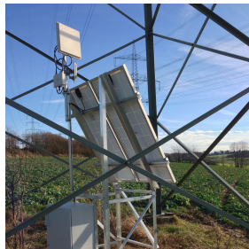
Build up at location A
